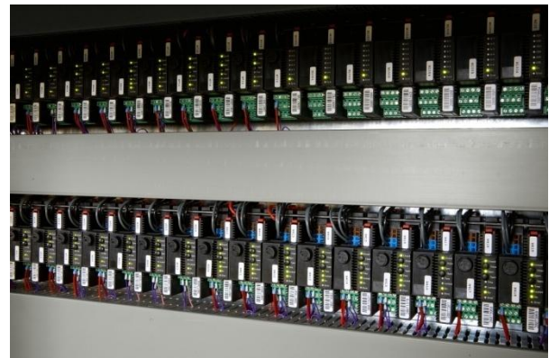
I/O wiring can be directly connected to terminals on the Base Module. No additional terminals are needed.
